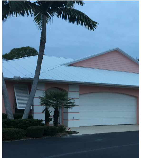
Examples of nearby homes with standing seam metal roofs
